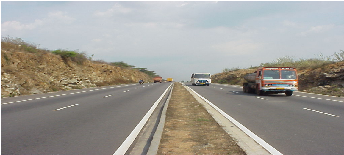
* Reduced Median with no earthen shoulders and no recovery zone in NH-7
