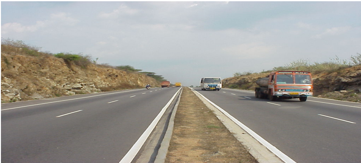
* Reduced Median with no earthen shoulders and no recovery zone in NH-7
