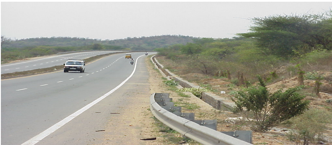
* "W" beam crash barrier does not provide any walking space and note open concrete drains at edge
